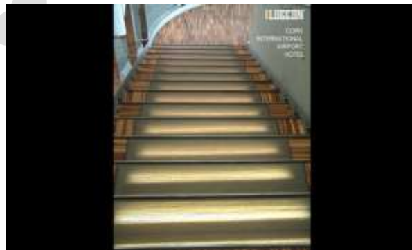
Fig.6. Translucent Concrete Stairs
