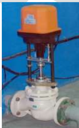
Fig.2 Electrically Actuated Control Valve
