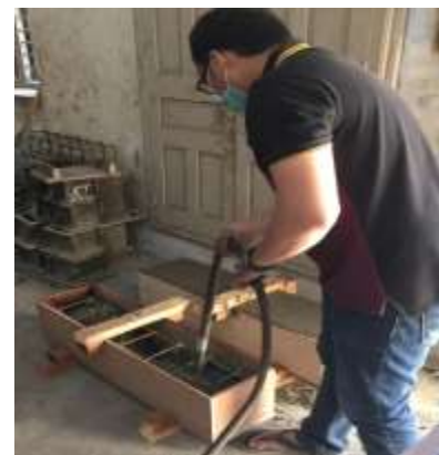
Figure 3: Casting of beam
