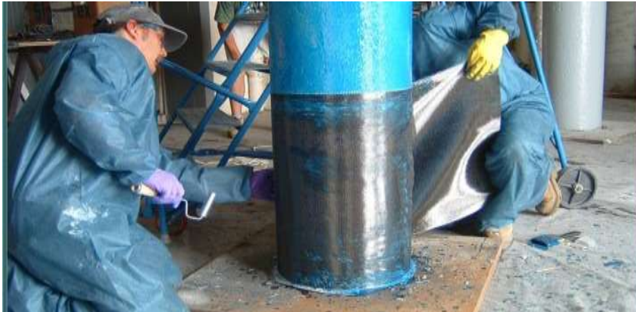
Fig.1.1.Jacketing of GFRP sheets around column
