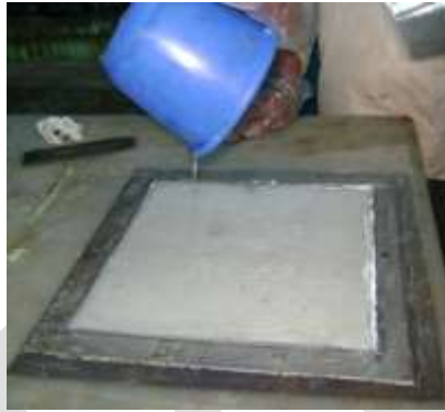
Fig -2: Pouring of Epoxy Resin
