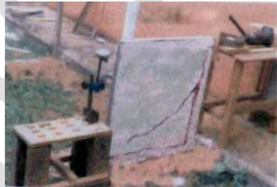
Figure 3: Failure Mode of MF1 Frame
