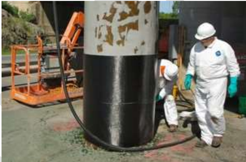
Fig.1.2..Jacketing of CFRP sheets around column
