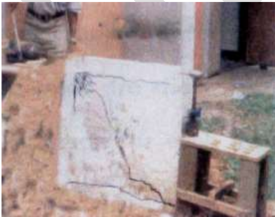
Figure 4: Failure Mode of MF2 Frame
