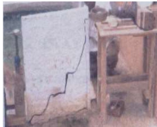
Figure 5: Failure Mode of MF3 Frame
